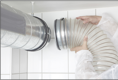
Fig 9: Connecting the hose to the duct to be cleaned
