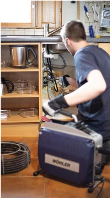
Fig. 13: Drain cleaning
