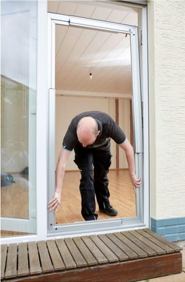
Fig. 19: Fitting the frame into the door cut-out
