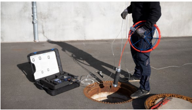
Fig. 71: Positioning the inflatable sealing bladder in the pipe
