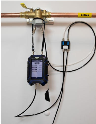
Fig. 25: Connections for leak tightness testing
