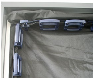
Fig. 18: Wide and narrow clamps positioned
