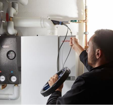
Fig. 12: Positioning the upper sealing bladder with telescope set and viper
