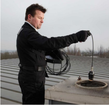
Fig. 5: Inspections using camera cable from above
