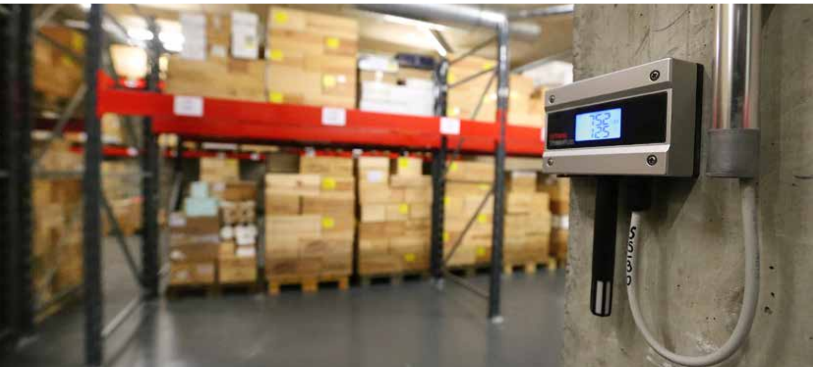
One of the 227 Rotronic HygroFlex transmitters in the duty-free warehouse of Ports Francs.
